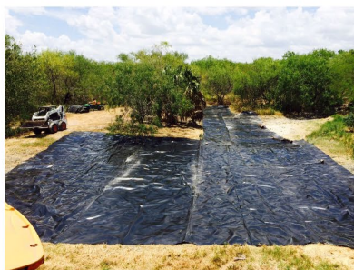
The expansion of wetlands involved clearing brushes, installing liners and pipes, and digging out ponds.
